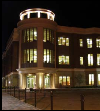
Ceramic Metal Halide on Façade with High Pressure Sodium Streetlights
